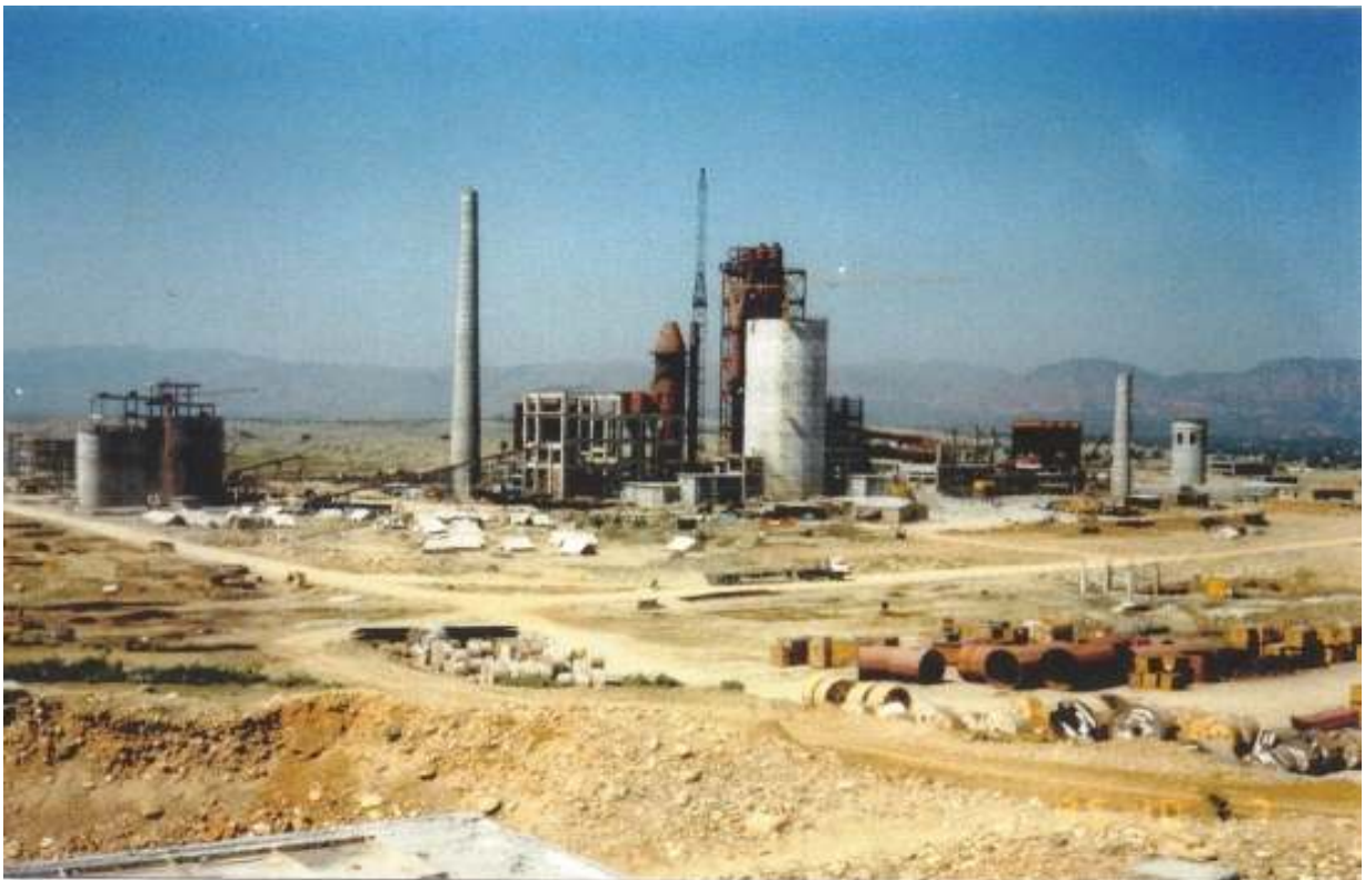
160 FEET HIGH BLENDING SILO AND 250 FEET HIGH CHIMNEY OF ARMY WELFARE TRUST CEMENT PLANT AT NIZAMMPUR COMPLETED IN 1997
