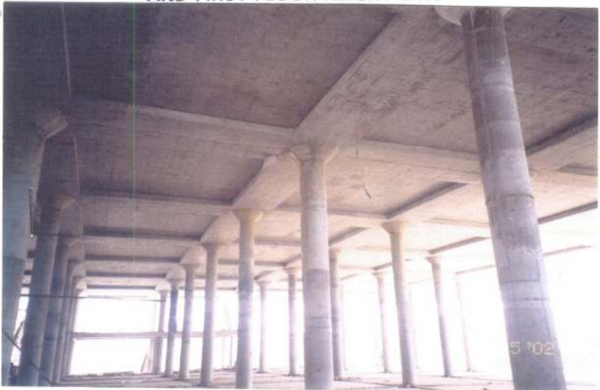
LUCKY TEX PRINTING BLOCK INTERIOR VIEW SHOWING 27ft COLUMN HEIGHT, COLUMN CAPITAL AND PANELLED SLAB FLOOR
