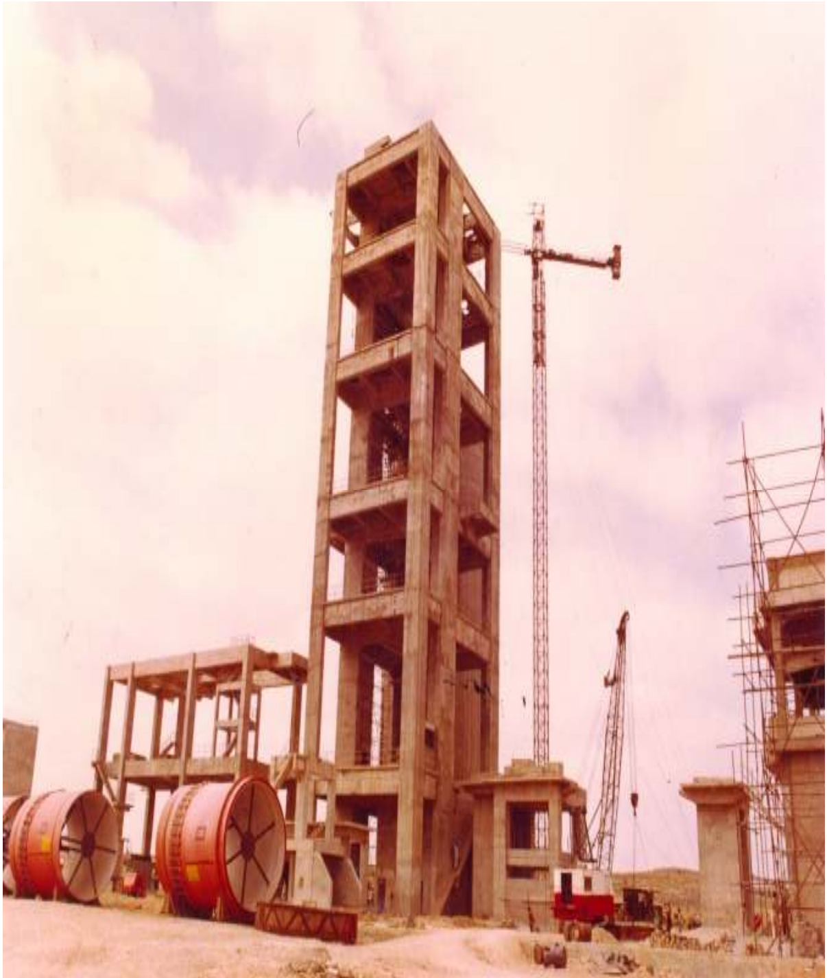
200 FT HIGH PREHEATED TOWER BUILDING OF PAKLAND CEMENT PLANT CONSTRUCTED IN 1983
