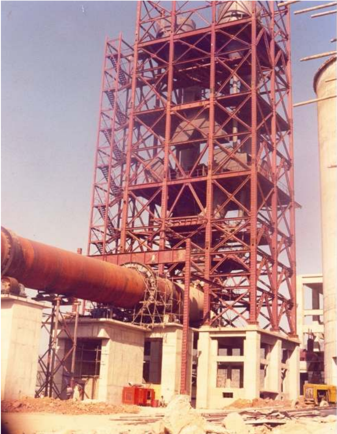
220 FEET HIGH PREHEATER TOWER IN STEEL AT FECTO CEMENT PLANT
