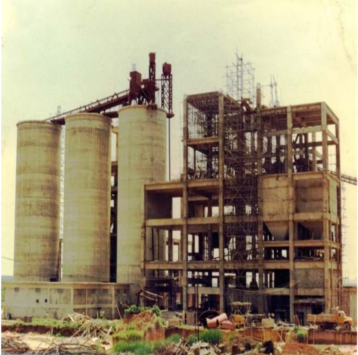
CEMENT SILO AND FINISH MILL OF 2000 TDP AT FECTO CEMENT PLANT
