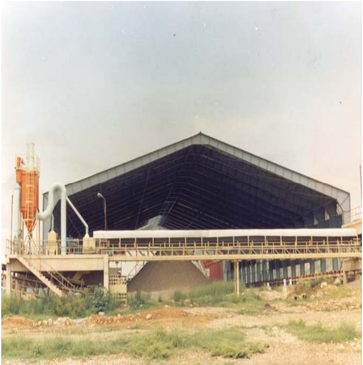
150 FEET SPAN BY 675 FEET LONG SHED OVER PREHOMGENISING BED FOR FECTO CEMENT PLANT AT RAWALPINDI AND PAKLAND CEMENT AT KARACHI
