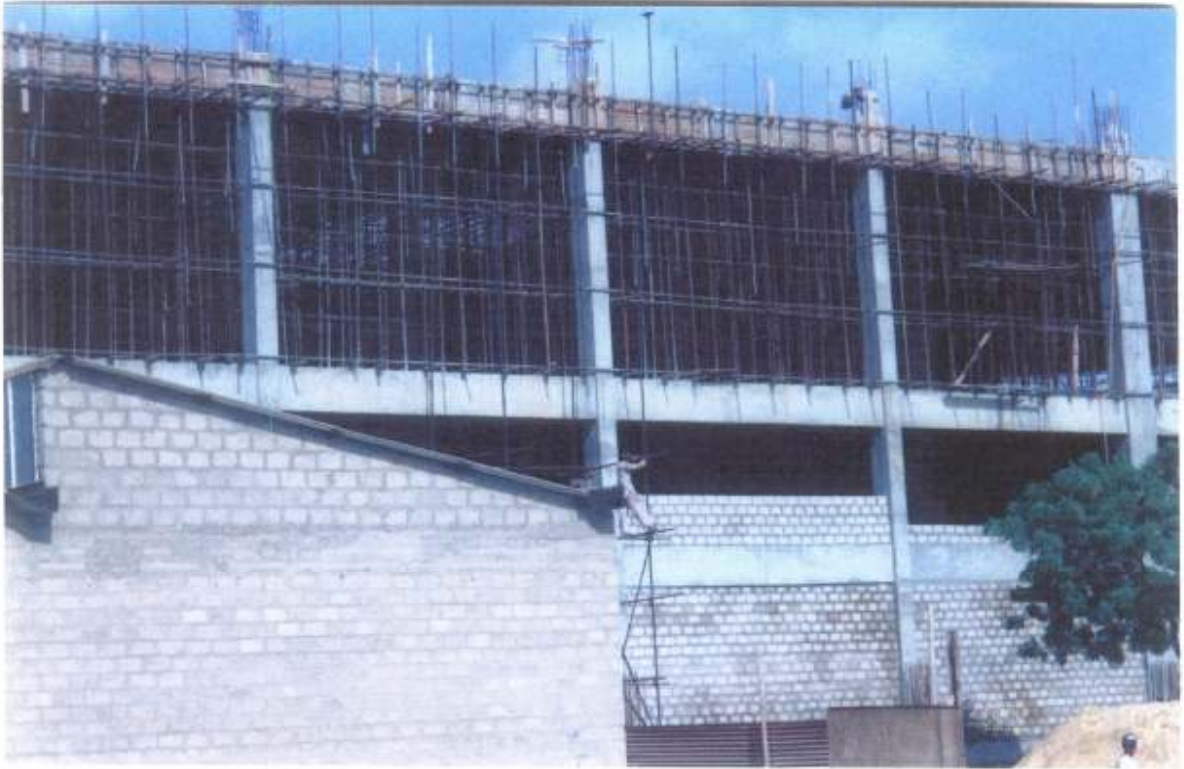
A VIEW OF LUCKY TEX. PRINTING BLOCK UNDER CONSTRUCTION NOTE:- GROUND FLOOR HEIGHT 27ft AND FIRST FLOOR HEIGHT 21ft
